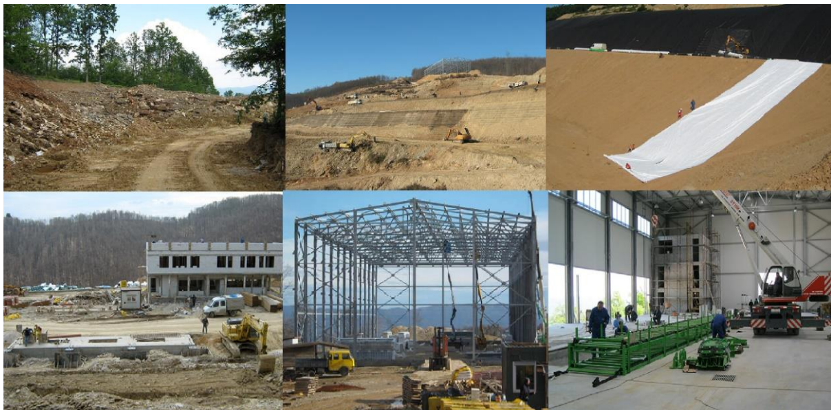
Figure 2 Overview over Duboko landfill construction
